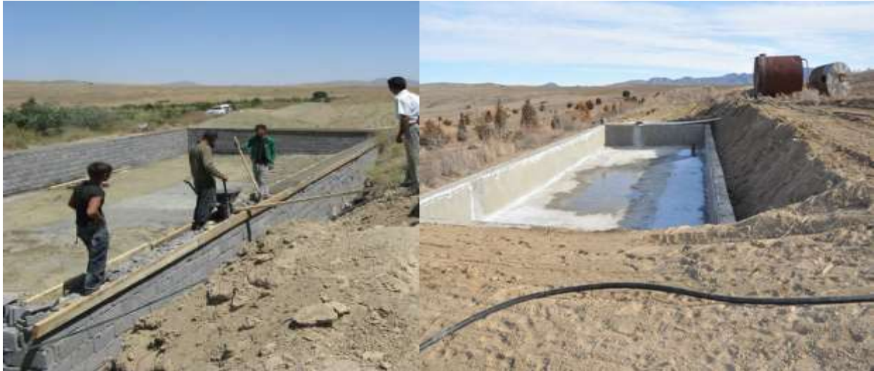
Construction of concrete basin (capacity - 400 m 3 ) for water storage
