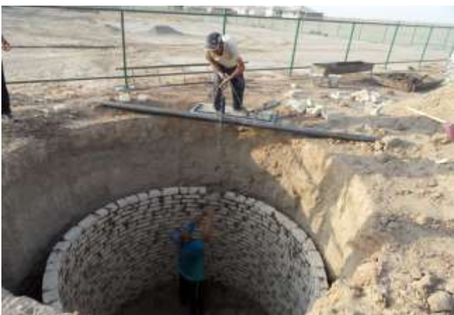
Construction of wells using the traditional method
