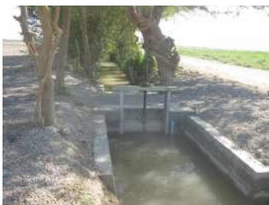
1. Construction of water regulating devices with one and two outlet/discharges
