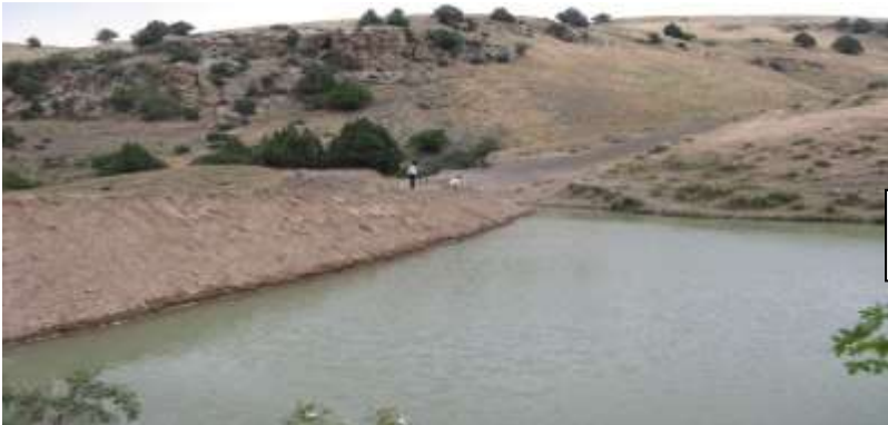
Construction of typical dam for water harvesting in Nohur
