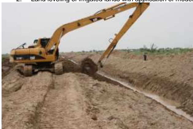
3. Reconstruction and cleaning of the inter-farm drainage collector
