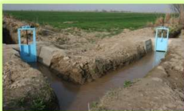
1. Construction of water regulating devices with one and two outlet/discharges
