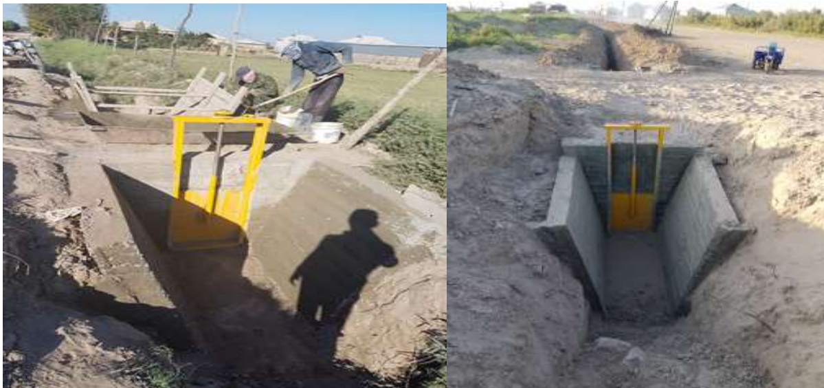
Digging ditch to deliver water from the canal to the village
